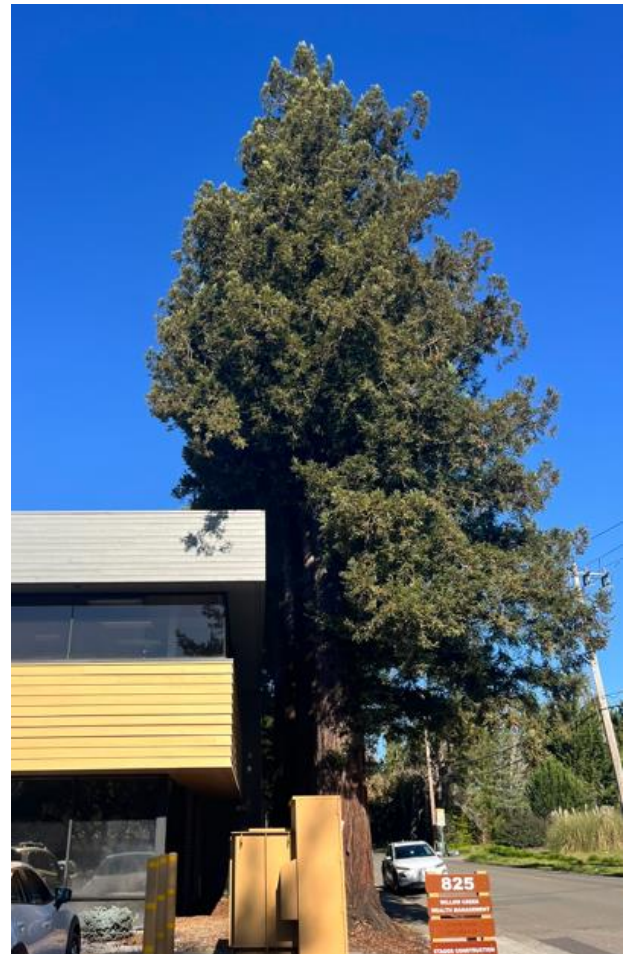
Figure 1. Subject trees viewed from the south showing how much of the canopy will need to be removed to provide total clearance above the roof and their proximity to the building and sidewalk.
