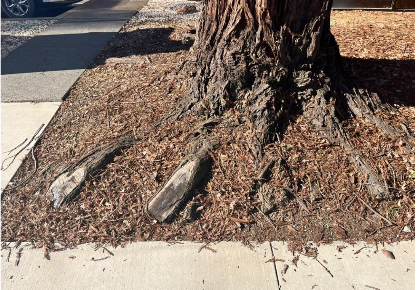
Figure 2. Cut roots and new sidewalk from the south-most tree. The sidewalk was almost certainly repaired due to lifting from the roots, which were almost certainly cut to perform the repair. These cuts may have destabilized the tree.
