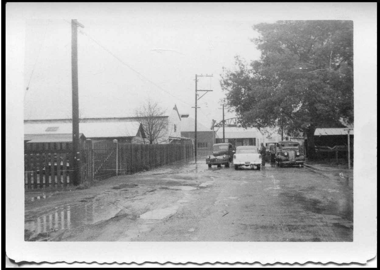
Figure 10 1951 at McKinley Street, which runs east-west behind both industrial structures and through the middle of the site. The building with light cladding and gable roof to the left of the cars is 6782 Sebastopol Avenue and the darker building with a hip roof and a conveyor bridge over the street is the real portion of 6780 Depot Street (Courtesy of the online photographic archives collections of the Western Sonoma County Historical Society, accessed via the Sonoma County Library).
