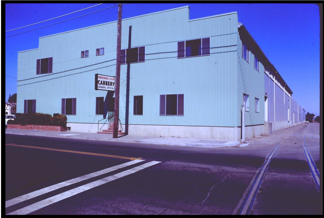
Figure 15 This 1970 photograph shows that original, circa 1924, fenestration and siding of the façade and side elevations of 6780 Sebastopol Avenue had been replaced with manufactured wood siding, known as T1-11 and fixed and sliding aluminum frame windows. Note that a contemporary sign of backlit plastic sign above the entrance reads "Sebastopol Co-op Cannery." (Courtesy of the online photographic archives collections of the Western Sonoma County Historical Society, accessed via the Sonoma County Library).
