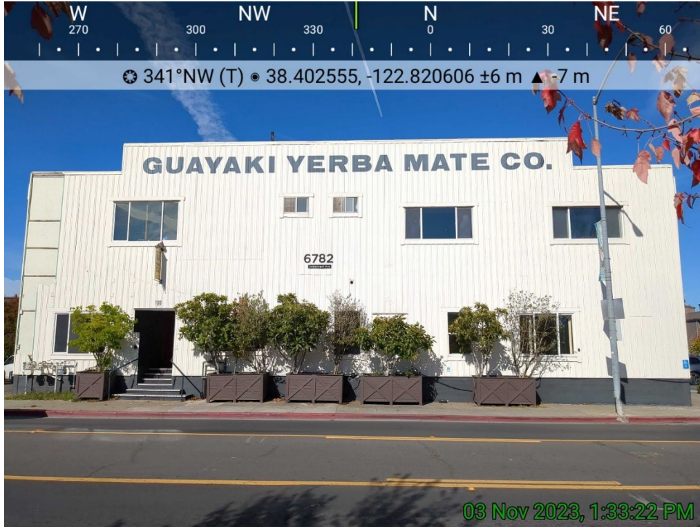
Figure 18 Façade with late-20th Century replacement siding, fenestration, and cornice cap (Photography by Yarbrough Architectural Resources 11/3/2023).
