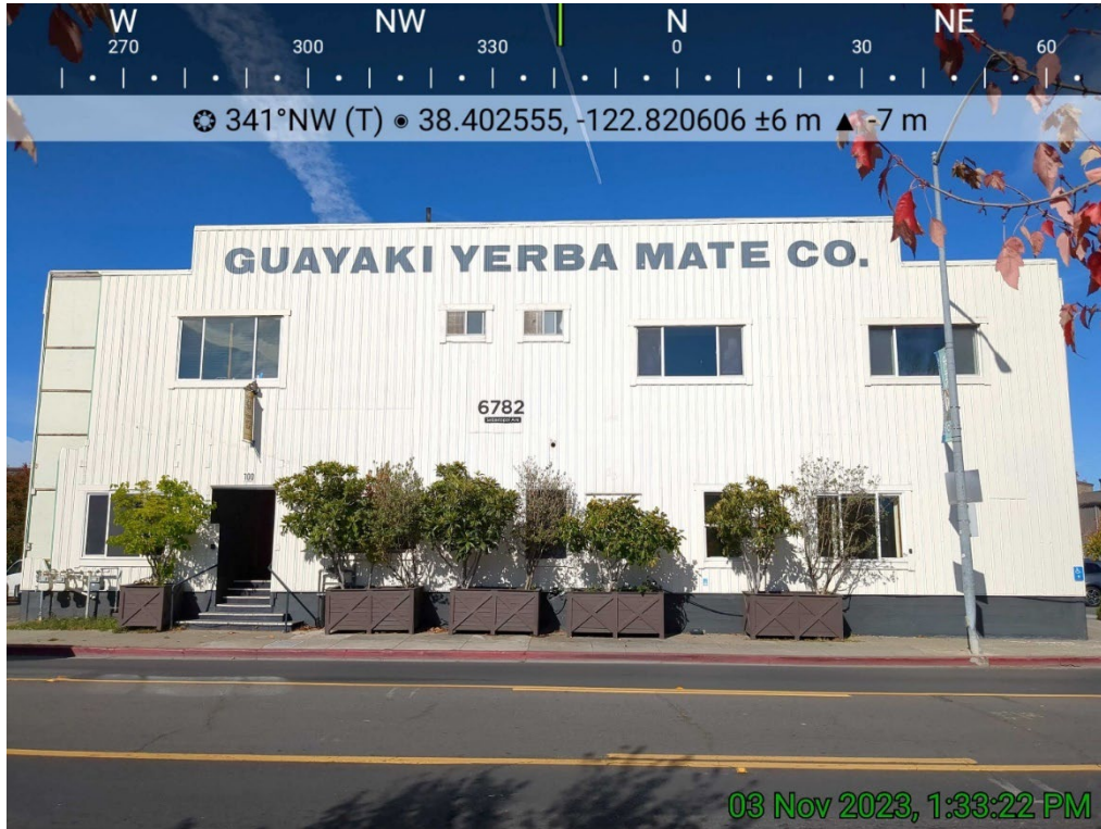
Figure 2 Façade with late-20th Century replacement siding, fenestration, and cornice cap (Photography by Yarbrough Architectural Resources 11/3/2023).
