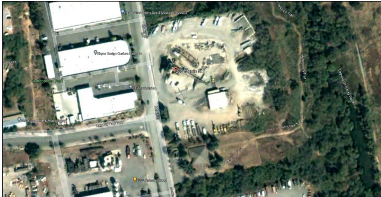
Photo 1. Historical aerial imagery of the Project Site, showing history of disturbance on the site, with active concrete plant. The oxbow wetland to the east of the Project Site is seasonally dry. Aerial imagery date: October 19, 2003.
