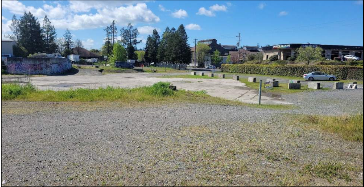
Photo 3. Overview of the Project Site, showing concrete pad, gravel/paved areas, discarded concrete blocks, and ruderal vegetation (Community 7). Facing south; photo taken April 5, 2024.
