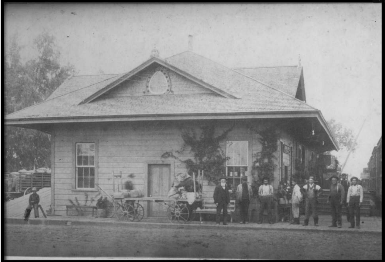
Figure 4 1905 depot on Depot Street, west of 6780 Depot Street (Courtesy of the online photographic archives collections of the Western Sonoma County Historical Society, accessed via the Sonoma County Library).
