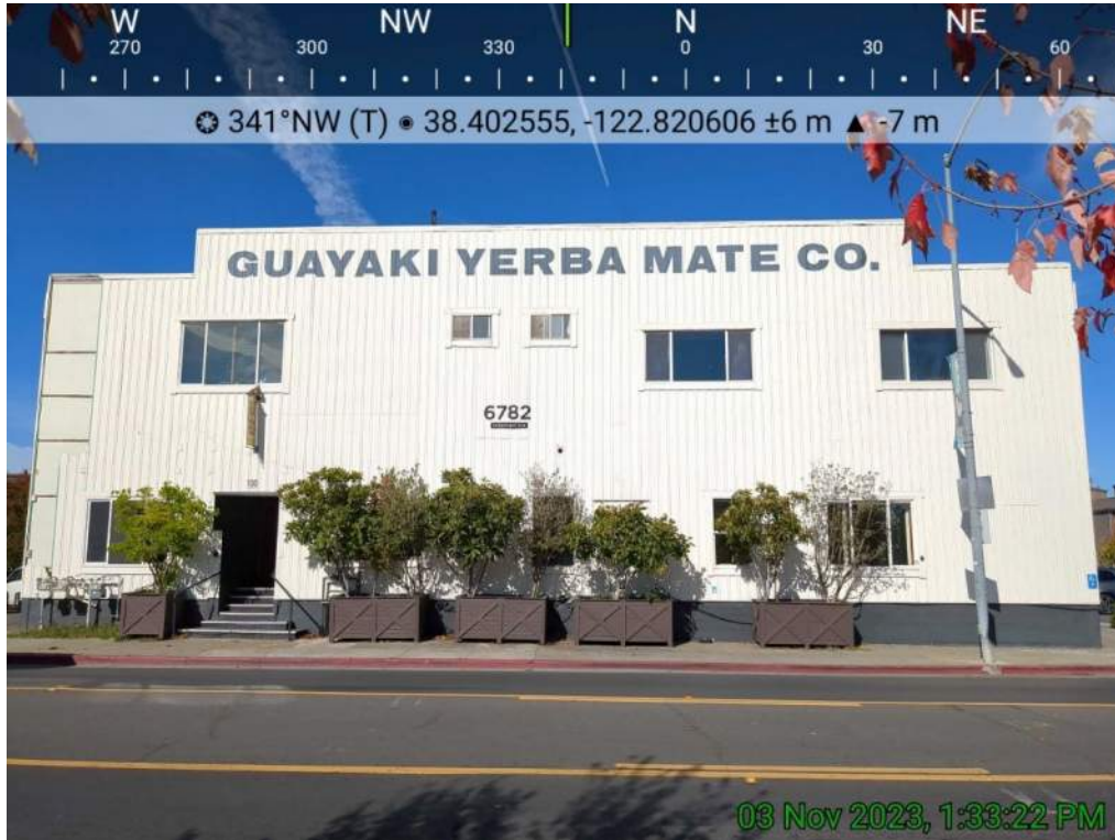
Figure 2 Façade with late-20th Century replacement siding, fenestration, and cornice cap (Photography by Yarbrough Architectural Resources 11/3/2023).
