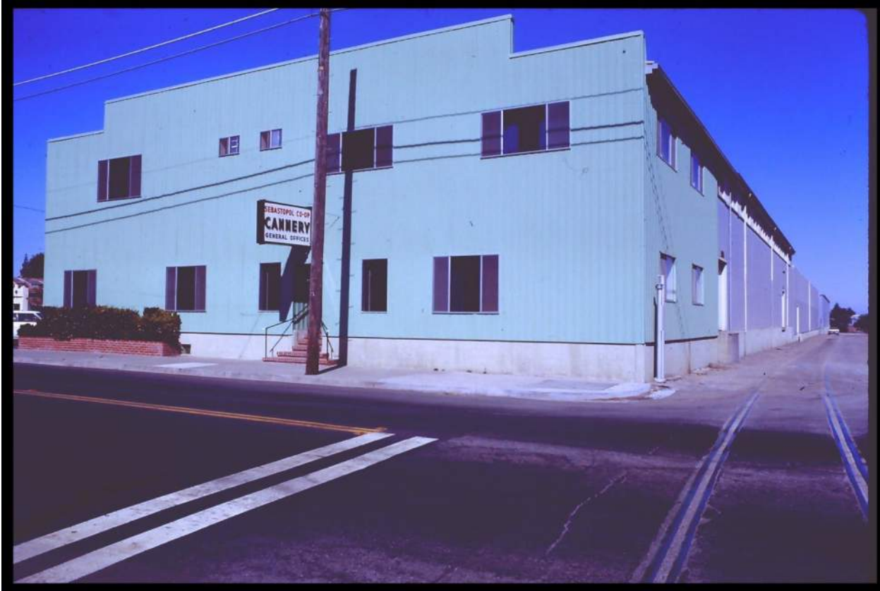
Figure 14 This 1970 photograph shows that original, circa 1924, fenestration and siding of the façade and side elevations of 6782 Sebastopol Avenue had been replaced with manufactured wood siding, known as T1-11 and fixed and sliding aluminum frame windows. Note that a contemporary sign of backlit plastic sign above the entrance reads “Sebastopol Co-op Cannery.” (Courtesy of the online photographic archives collections of the Western Sonoma County Historical Society, accessed via the Sonoma County Library).
