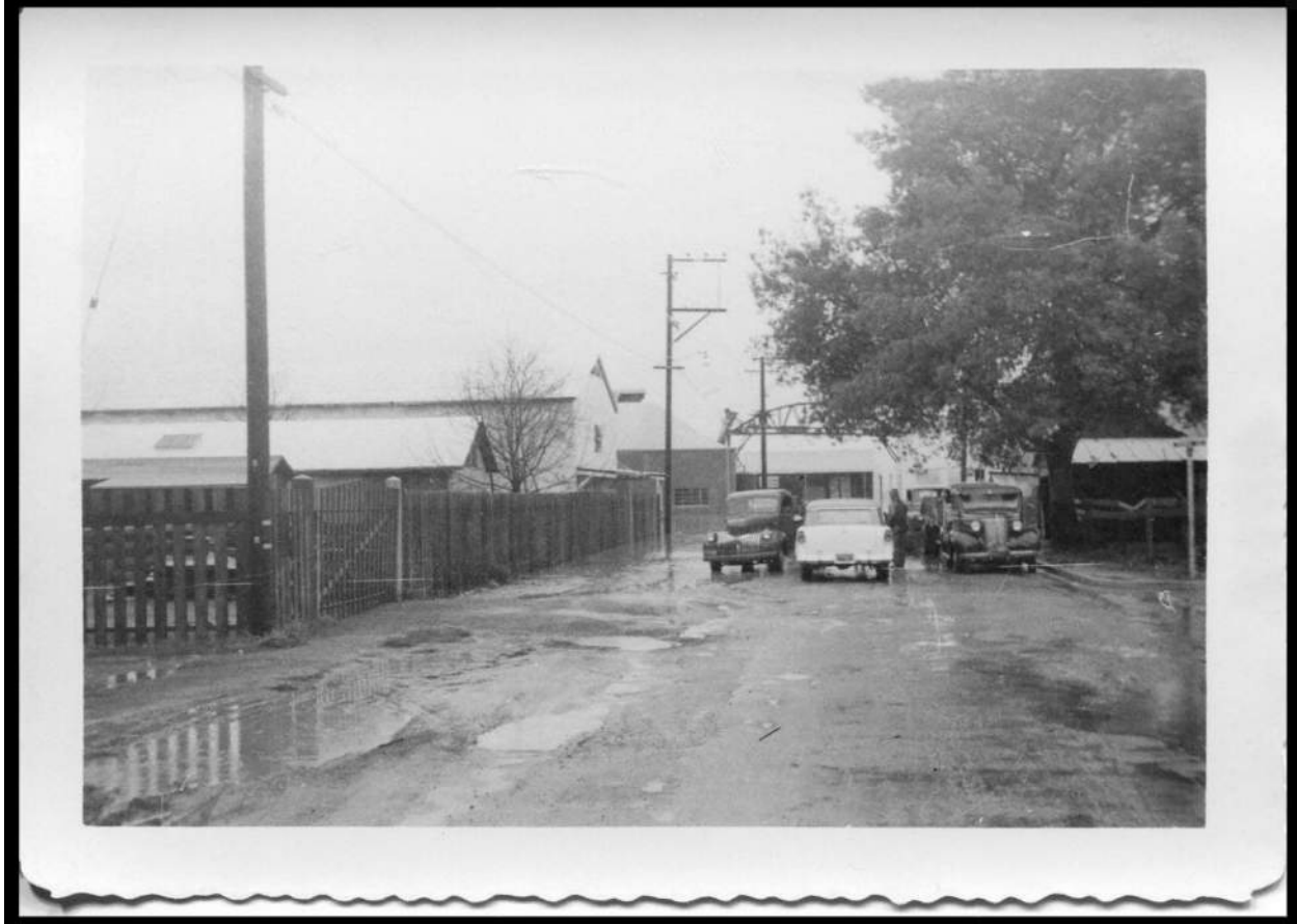
Figure 10 1951 at McKinley Street, which runs east-west behind both industrial structures and through the middle of the site. The building with light cladding and gable roof to the left of the cars is 6782 Sebastopol Avenue and the darker building with a hip roof and a conveyor bridge over the street is the real portion of 6780 Depot Street (Courtesy of the online photographic archives collections of the Western Sonoma County Historical Society, accessed via the Sonoma County Library).
