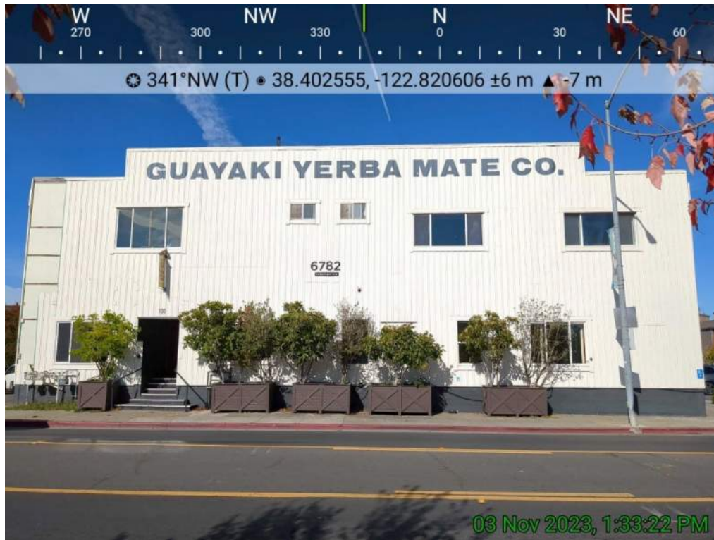
Figure 18 Façade with late-20th Century replacement siding, fenestration, and cornice cap (Photography by Yarbrough Architectural Resources 11/3/2023).
