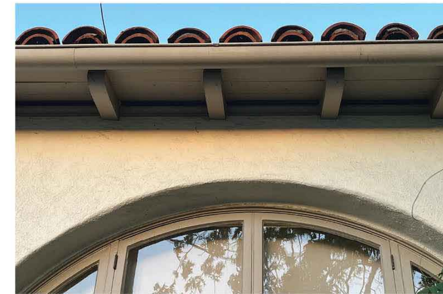
Painted Wood Rafters
