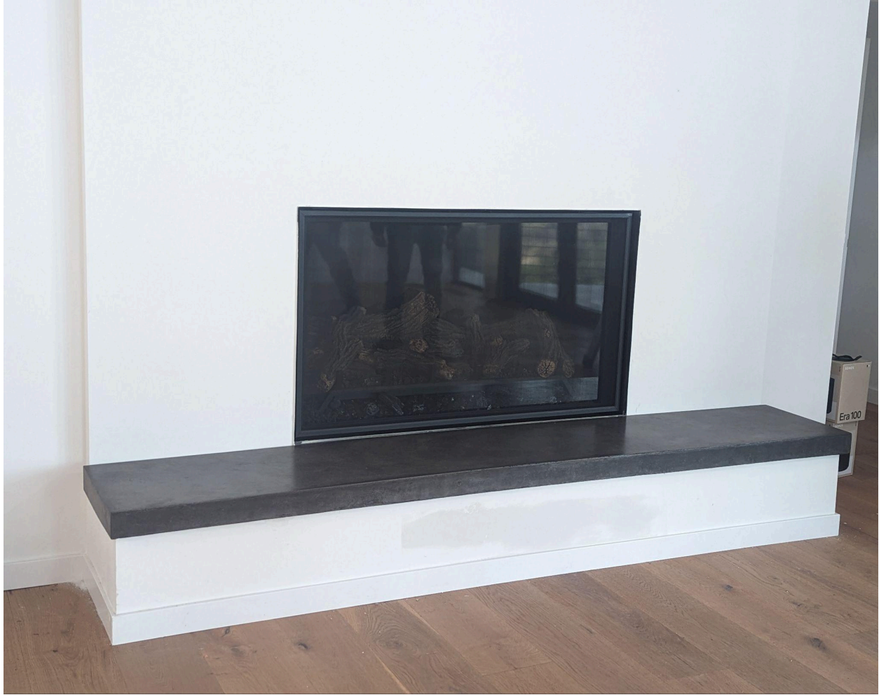
By Ryder Holmes Wilson. 20" x 104" gray pigmented concrete hearth for Les Milles house in Sebastopol, CA in 2023. Two hearths commissioned for $2900. Contact: Alex Richter, 707 338 1627
