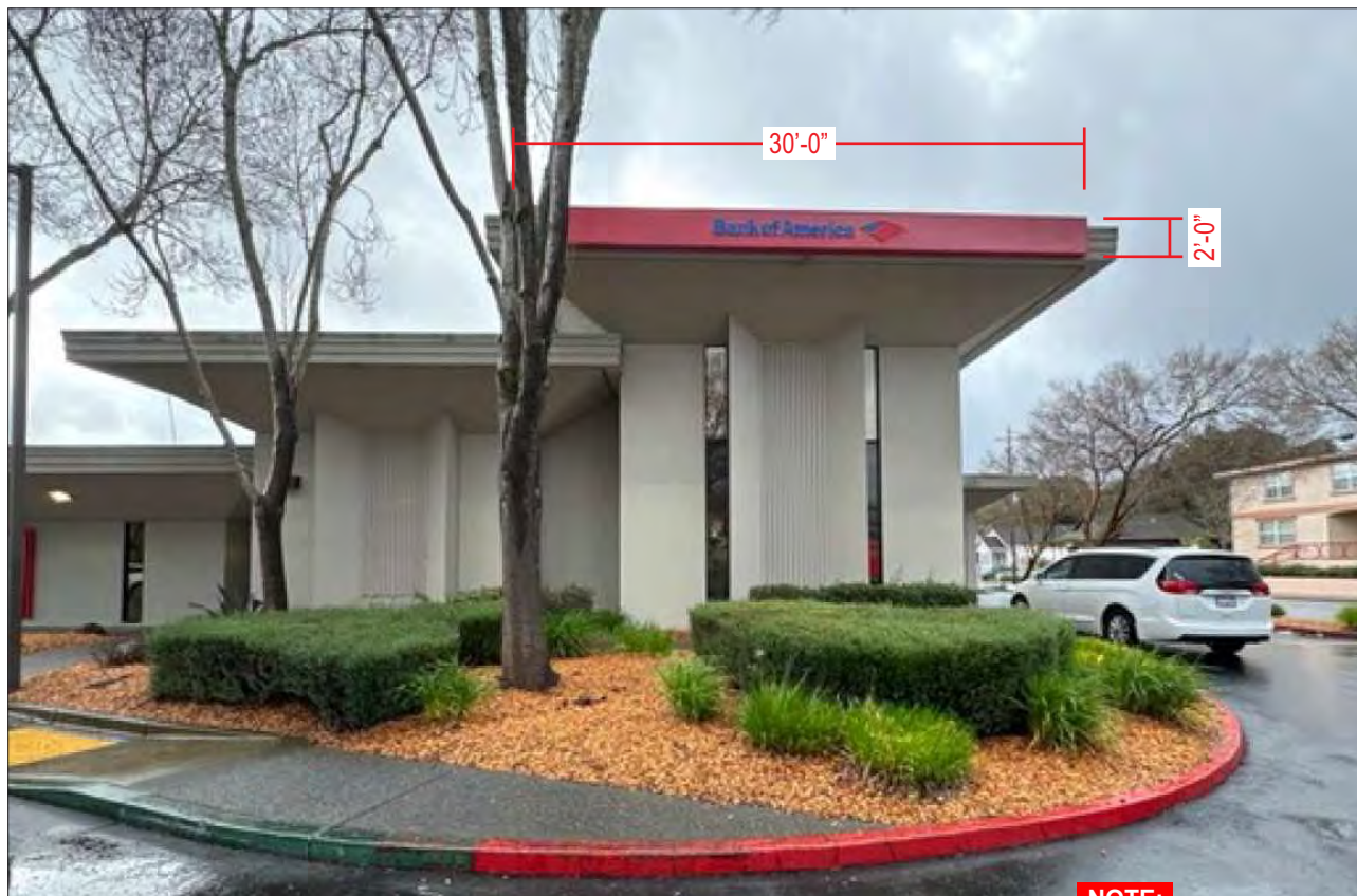
PHOTO SURVEY OF EXISTING Scale: 3/32" = 1'-0"
