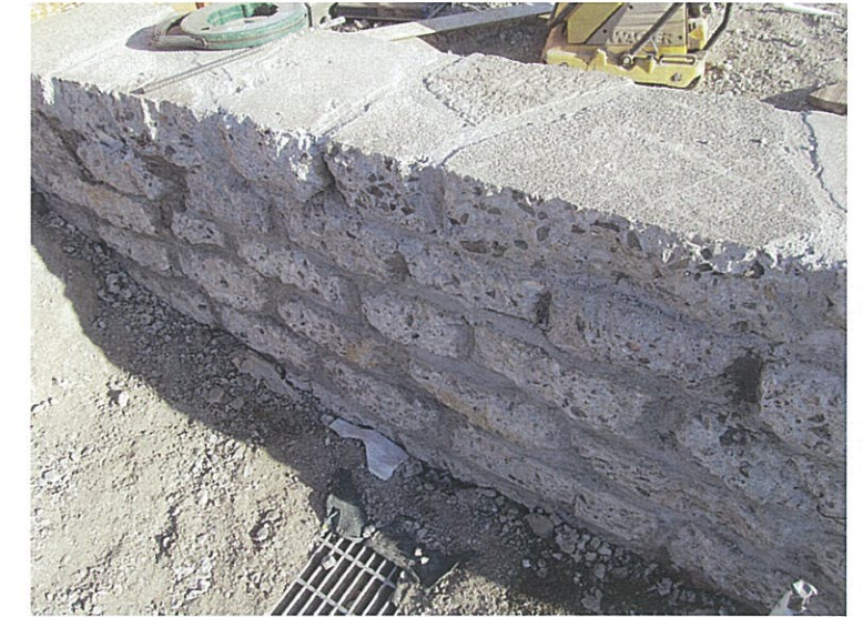
RECLAIMED CONCRETE WALL
