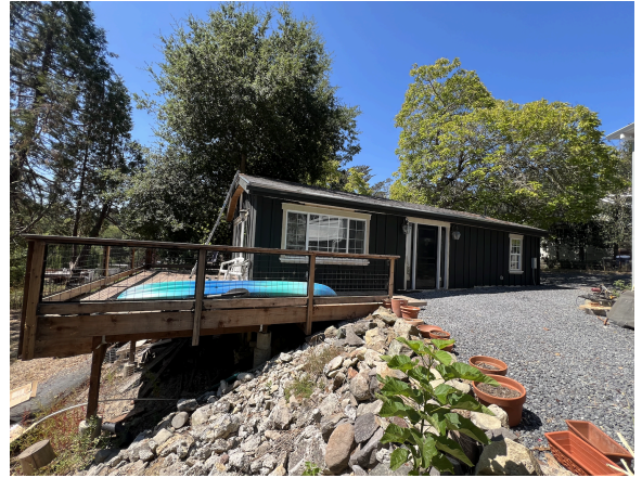
6. North/East Facing Side; showing deck
