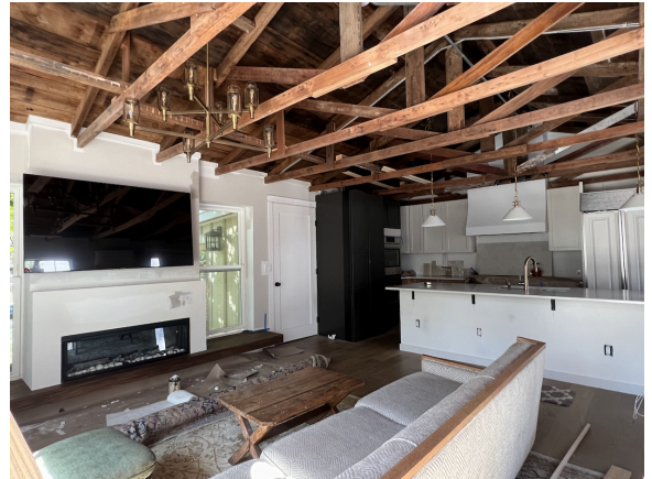
4. Towards Kitchen & Primary Bedroom
