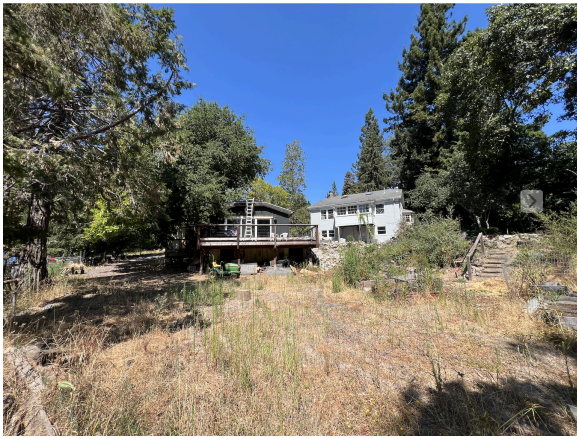
7. South/East Facing Deck; (ADU Left, Main House Right)
