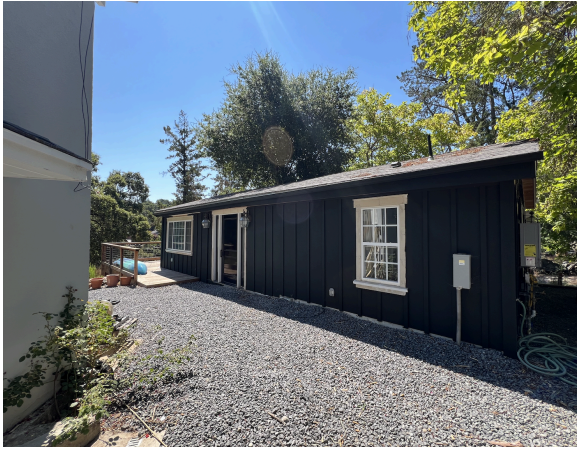
5. North/East Facing Side: Entrance of ADU
