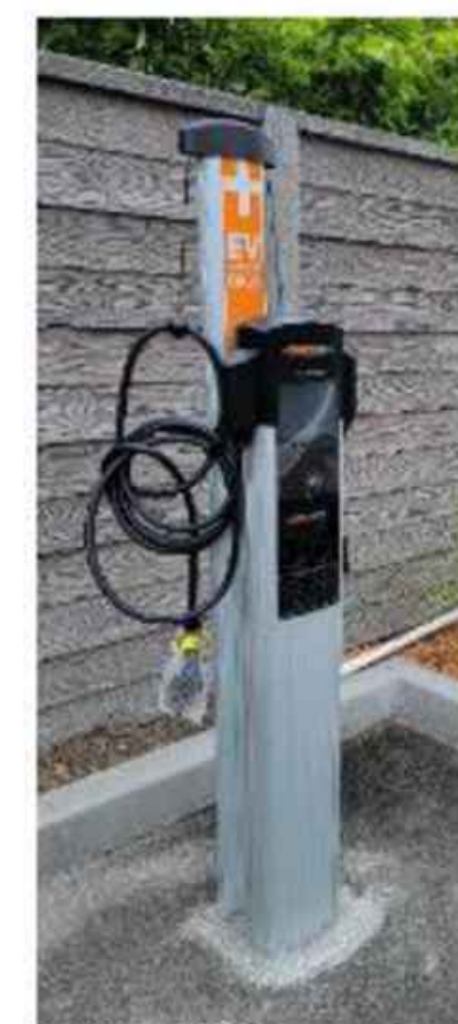
ELECTRIC VEHICLE CHARGING STATION -DOUBLE-SIDED
