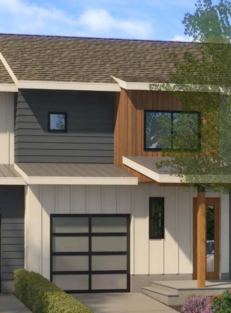
Hardie Board & Batt + Hardie Plank, Woodtone Summer Wheat Vertical Siding, Weathered Wood GAF Roofing
