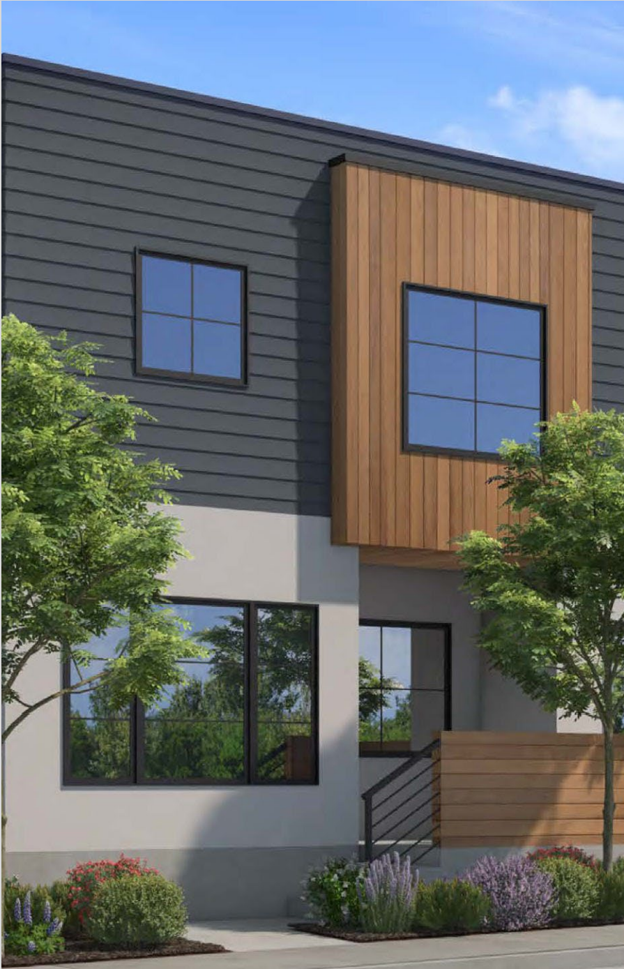
Hardie Plank, Stucco, Woodtone Summer Wheat Vertical Siding, Cedar Plank Deck Fencing
