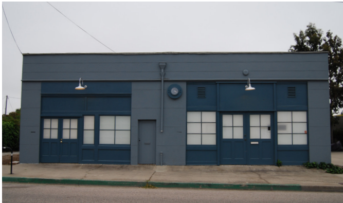
Example of a Maker Shopfront
