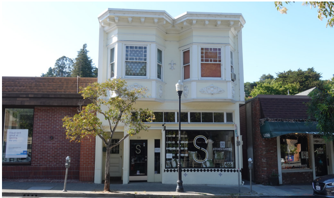
Example of Main Street Building
