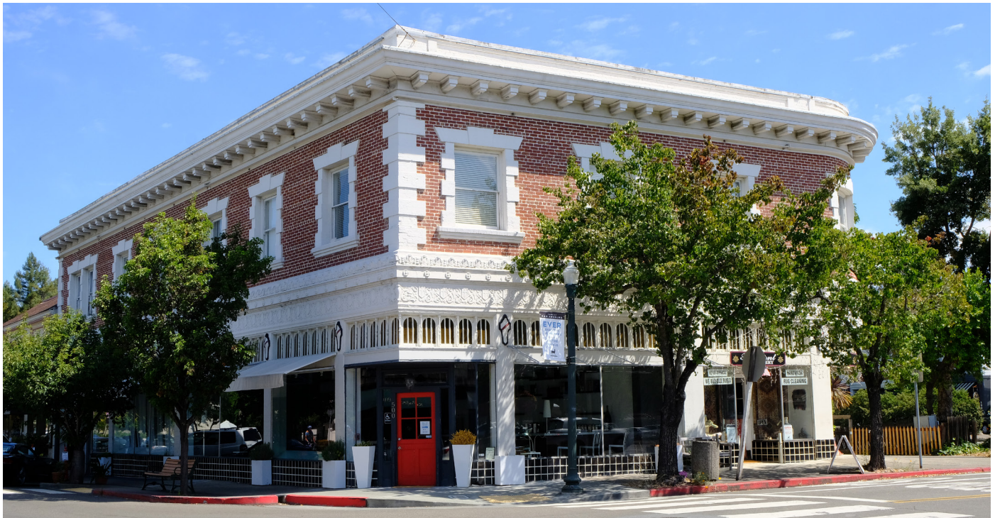
Example of Main Street Building
