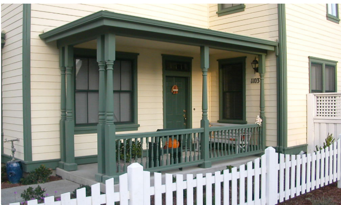
Example of an Engaged Porch
