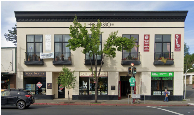
Example of Main Street Building
