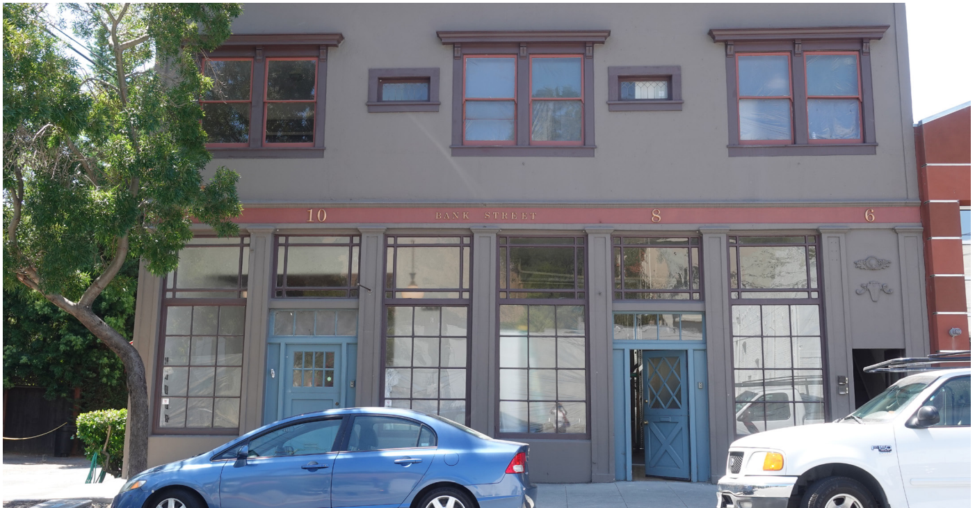
Example of a Maker Shopfront
