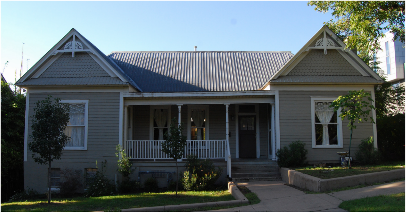
Example of an Engaged Porch
