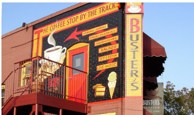
Example of Painted Wall Sign at a second story
