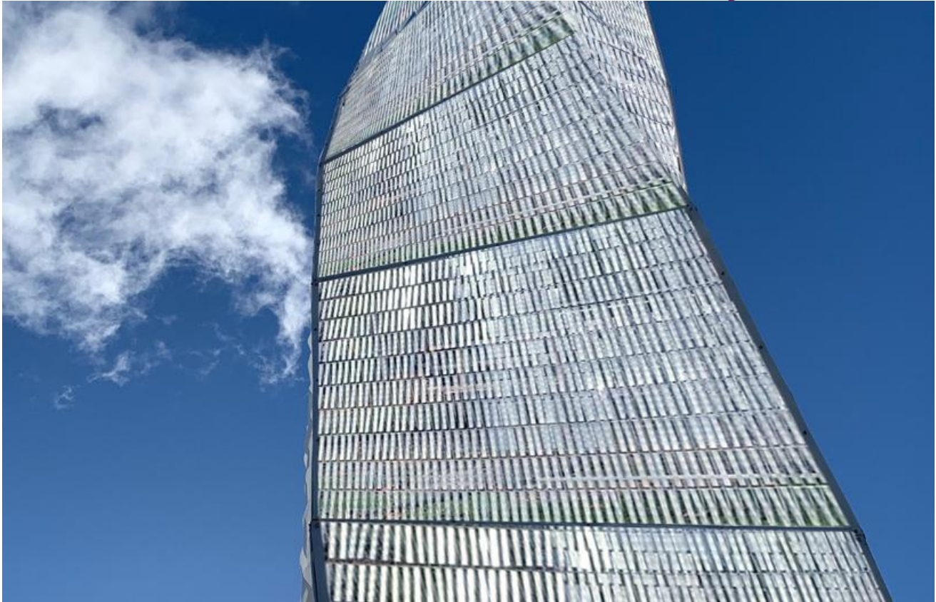
Detail of Column
