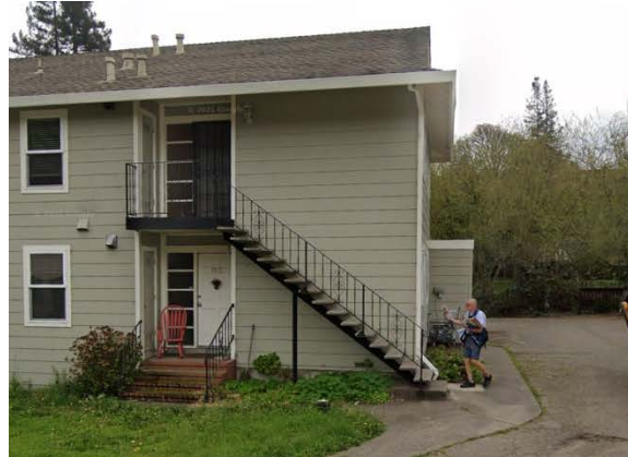
Example of Stoop covered by 2 nd floor stairs
