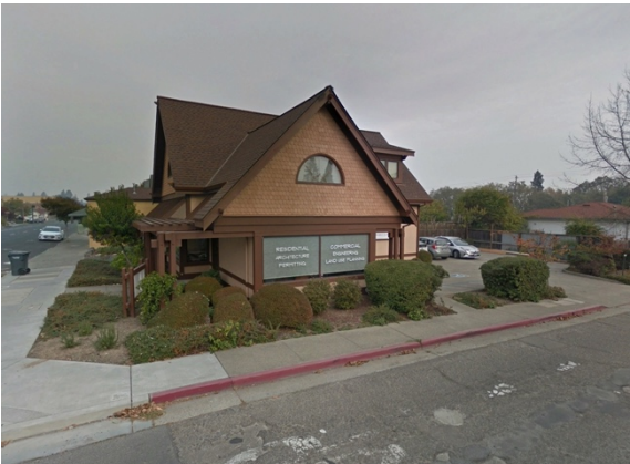
Example of office building on Petaluma Ave
