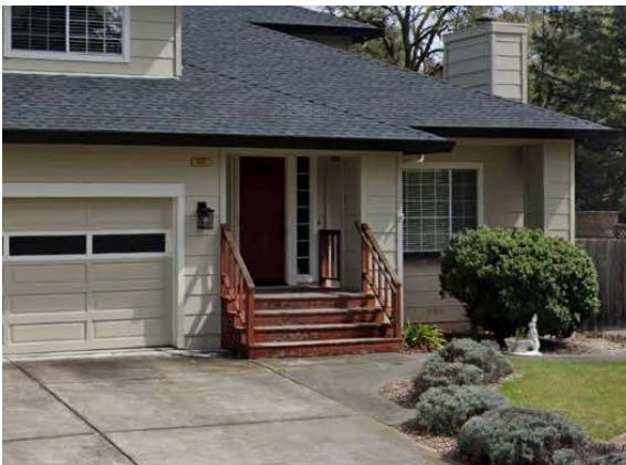
Example of raised, covered entry
