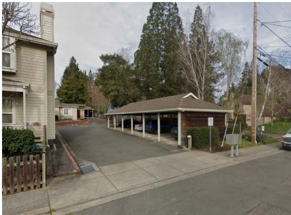
Example of detached carport at side of building
