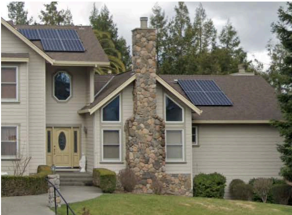
Example of chimney with stone veneer
