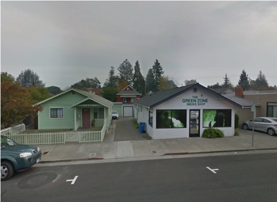
Example of side driveway to rear parking area
