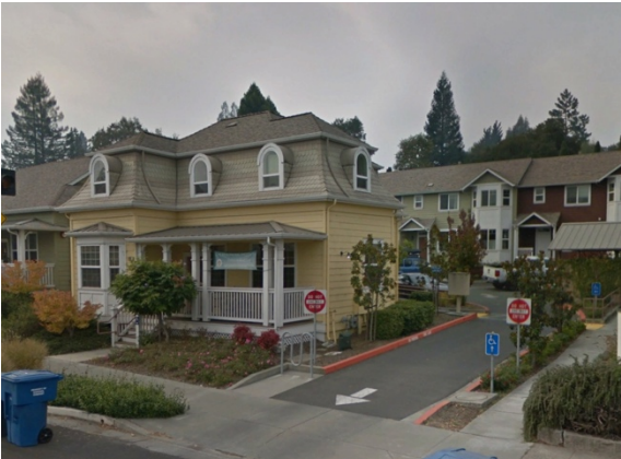
Example of commercial uses in converted houses in front and residential buildings in rear on S. Main St
