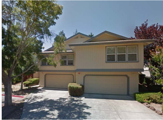
Example of Side-by-Side Duplex on Flynn St
