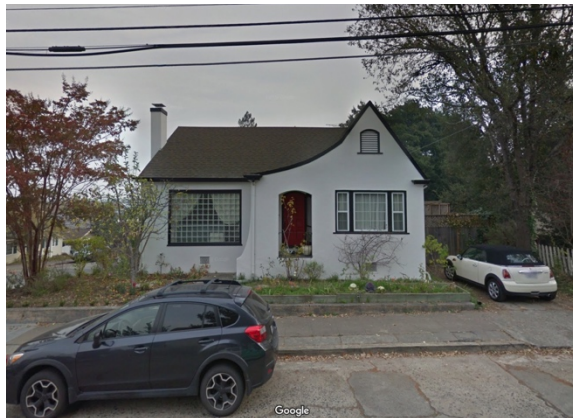
Example of Single-family house on S High St
