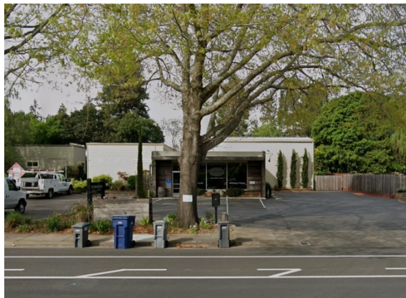
Example of office building on Gravenstein Hwy N
