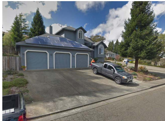
Example of garage at Side Street on Hawthorne Ct
