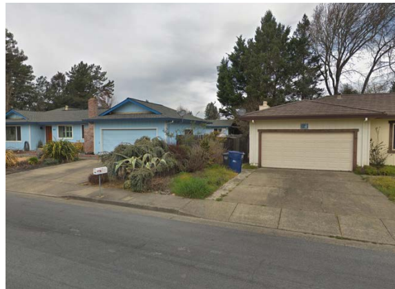
Example of garages on front façade on Hansen Ln
