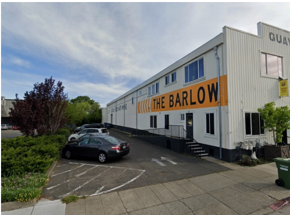
Example of parking along side of building
