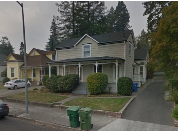
Example of Single-family house on S Main St
