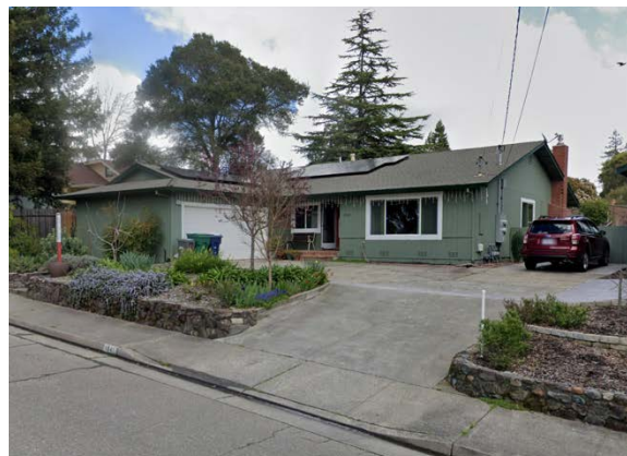
Example of a Single-family house on McFarlane Ave
