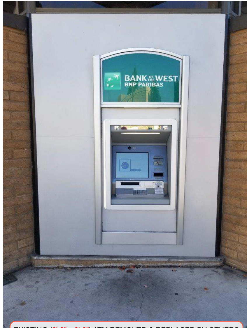
EXISTING (6'-3" x 3'-9") ATM REMOVED & REPLACED BY OTHERS
