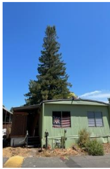
Photos #1 & 2: Front (South side) of 6850 Redwood - Looking North
