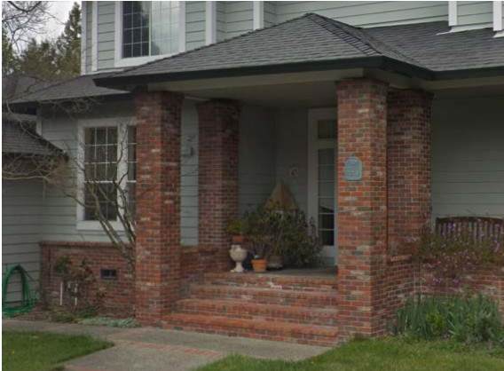
Example of raised, covered entry with brick
