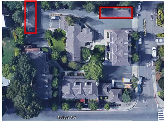
Aerial view of grouped parking in detached carports
