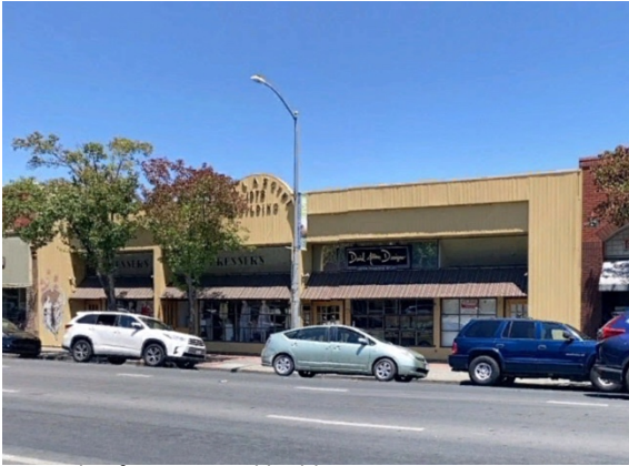
Example of Commercial building on N Main St
