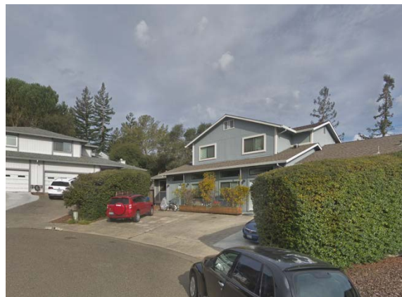
Example of parking spaces between the building and street
