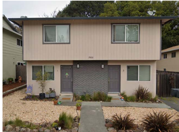
Example of ground floor with brick and stucco; upper story with siding
