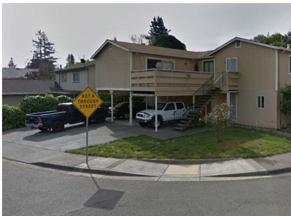
Example of parking spaces at Front Street
