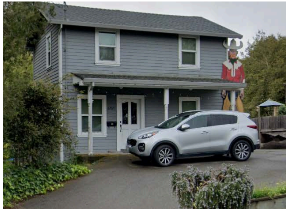
Example of Covered Entry
