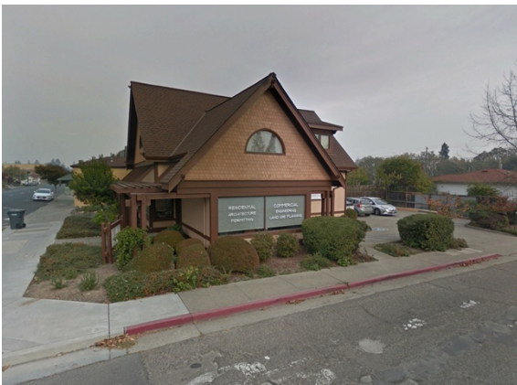
Example of office building on Petaluma Ave
