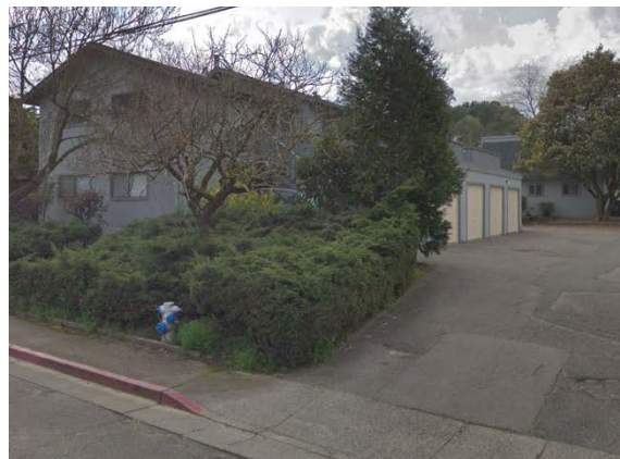
Example of attached garage at side of building
