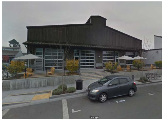
Example of metal panel wall cladding
