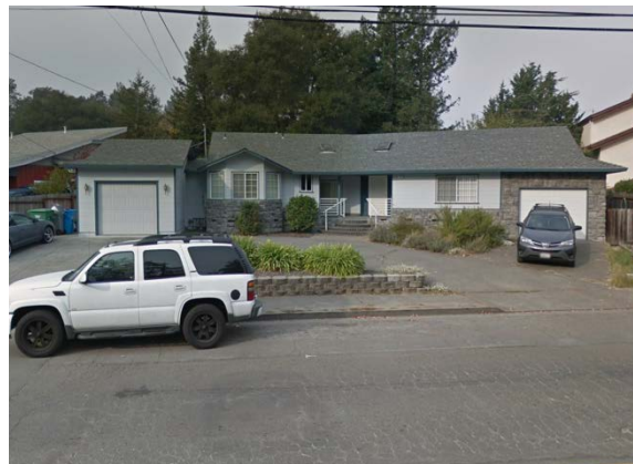
Example of Side-by-Side Duplex on Jewell Ave
