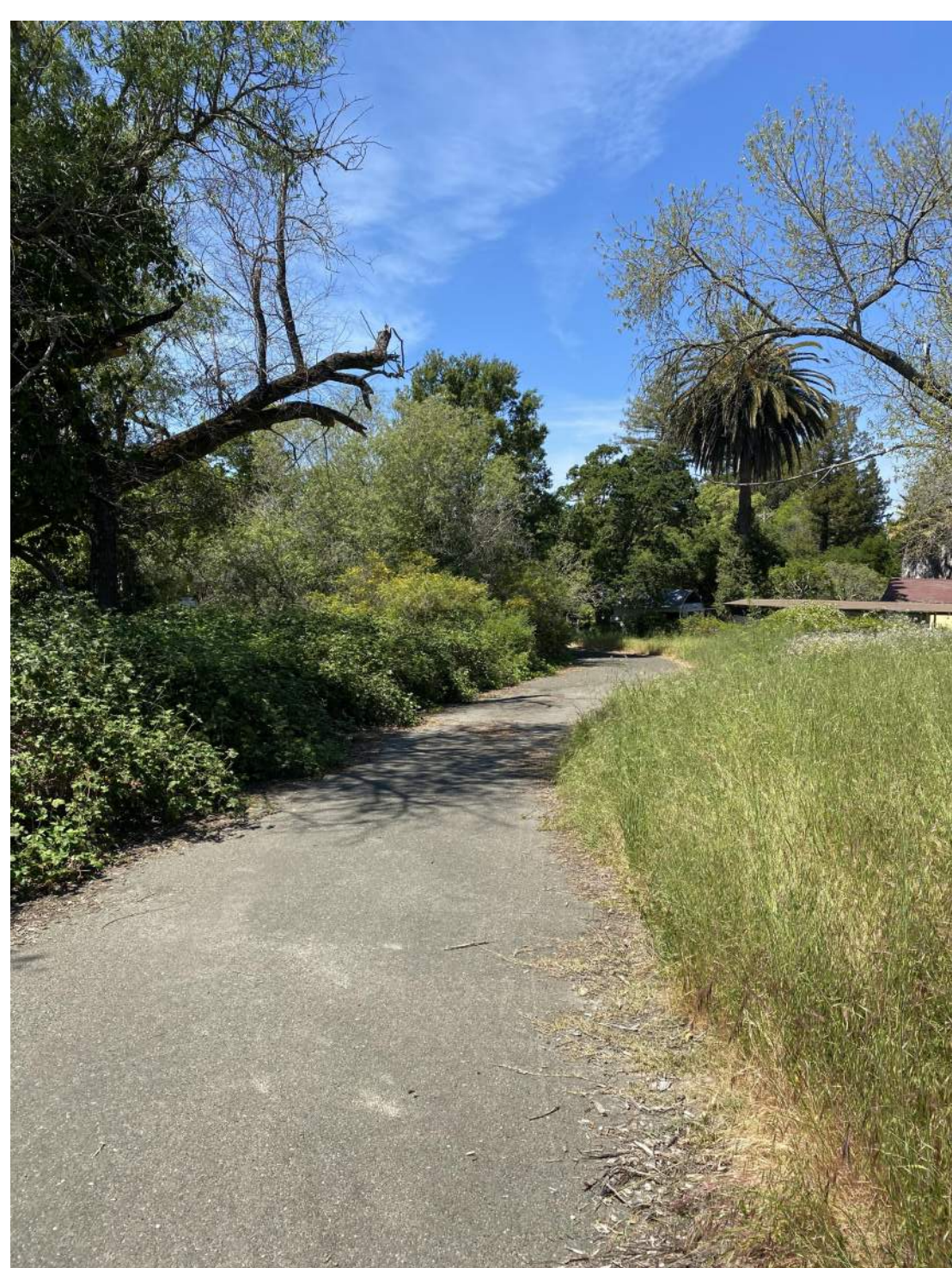
6 EXISTING ASPHALT DRIVEWAY (NORTH)
