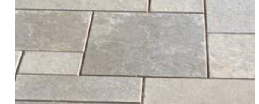
'Road' TILE at steps and porch decks
