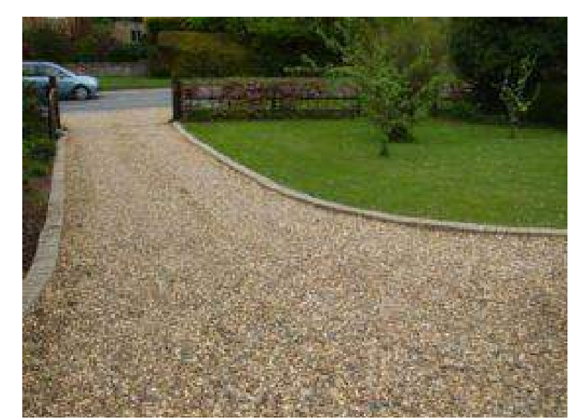
ADU DRIVEWAY 3/8" ANGULAR CRUSHED GRANITE W/ EDGE
