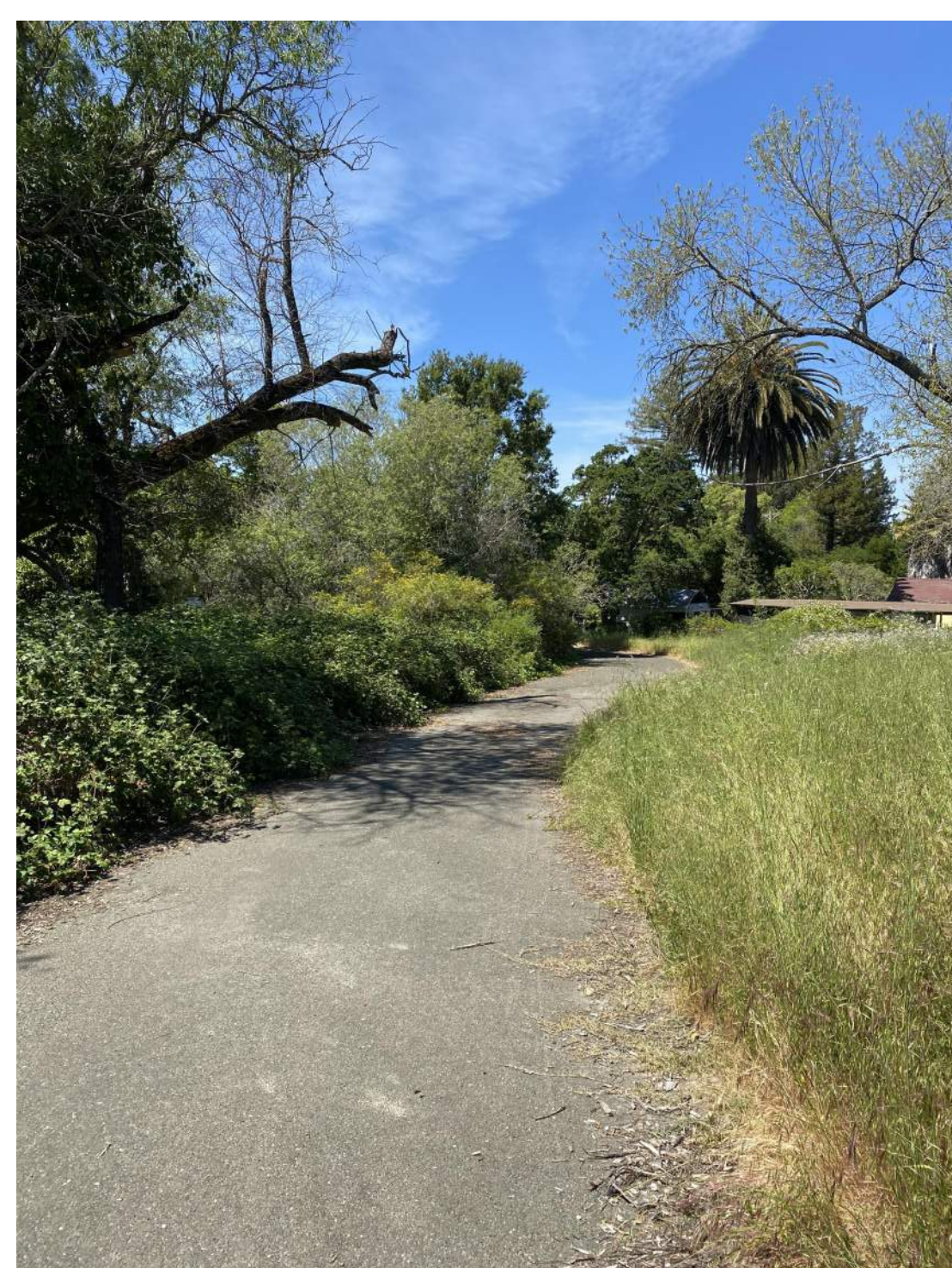
6 EXISTING ASPHALT DRIVEWAY (NORTH)
