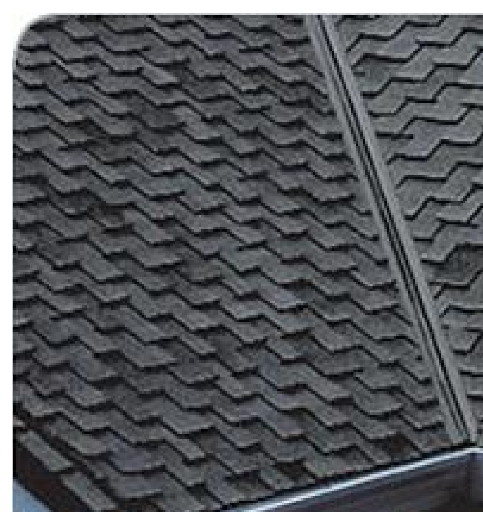
H ROOFING - Asphalt Shingle Dark Grey w/ 'Architectural' Shingle
