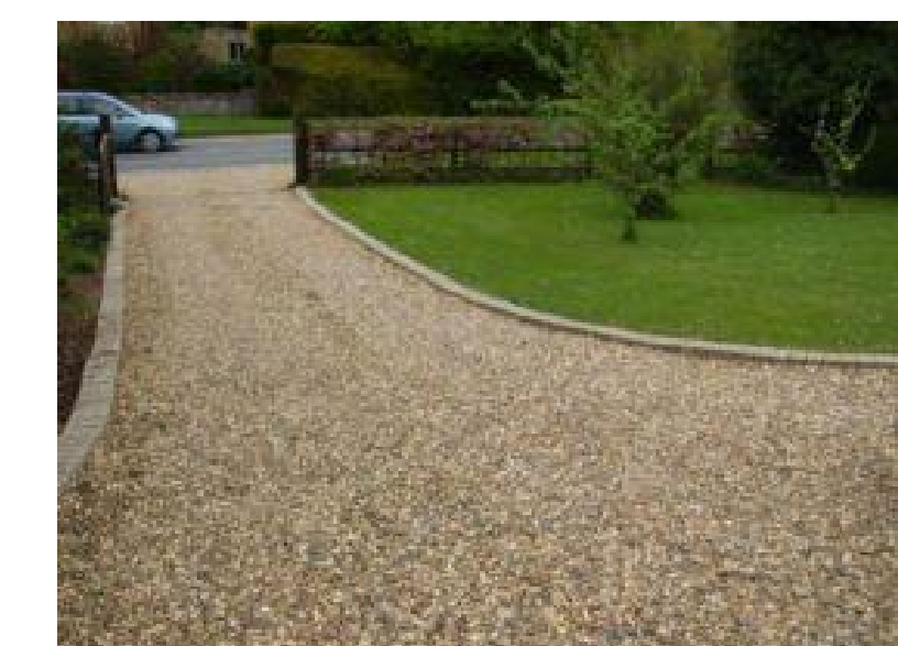
ADU DRIVEWAY 3/8" ANGULAR CRUSHED GRANITE W/ EDGE
