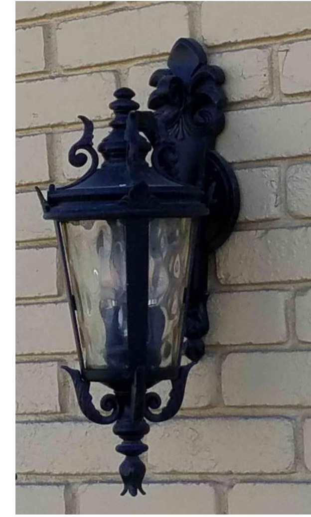
1E EXTERIOR LIGHT FIXTURE W/ TESLAR OR EQUIVELANT LED BULB 4.5 WATTS (3) PER FIXTURE
