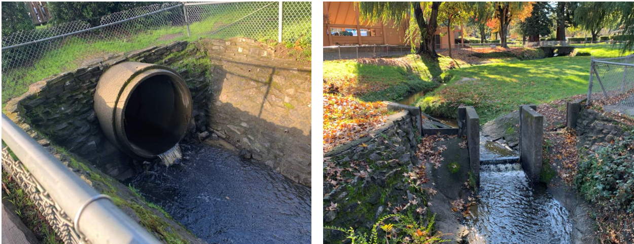
Figure 3 Left: Calder Creek at upstream end of Ives Park (looking toward the southwest); Right: Calder Creek at the central flashboard weir system within the heart of Ives Park.
