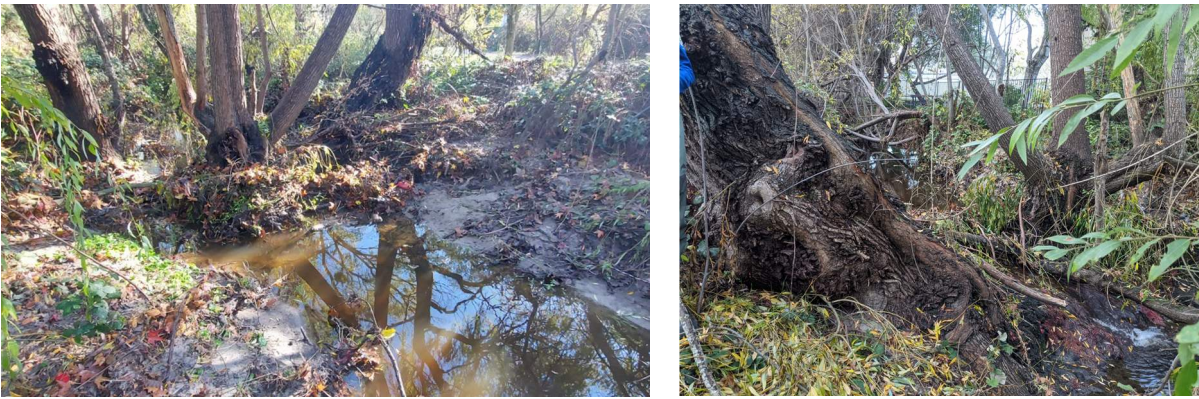
Figure 6 Non-native Mayten trees in Calder Creek channel approximately 125 ft downstream of the storm drain outfall. Rootwad obstruction causes approximate 1.7' drop in the bed elevation.
