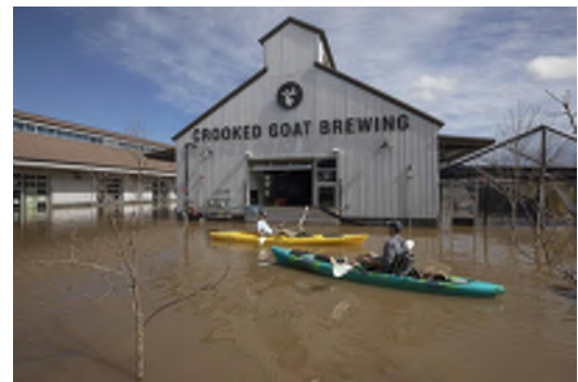
In February 2019, several businesses in The Barlow shopping district suffered from flooding after an atmospheric river stalled over the Russian River Watershed. An estimated two-thirds of the shopping district was flooded, including Park Village, a City-owned low income housing site, and the Community Cultural Center located on Morris Street. Photo Credit: John Burgess/The Press Democrat
