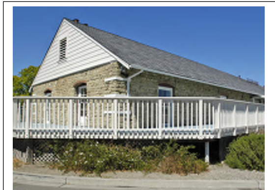
The Petaluma and Santa Rosa Railway Powerhouse is one of example of a historic place in Sebastopol. From its initial settlement in 1812 to the development of the railroad in 1870, Sebastopol and Sonoma County were dependent on horse and wagon for transportation. This powerhouse, and the wooden passenger depot at the West County Museum were constructed in 1902. Source: NRHP 2020
