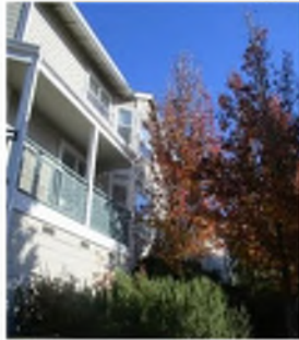
#1173 Gravenstein Hwy South (second level currently separate residential unit)
