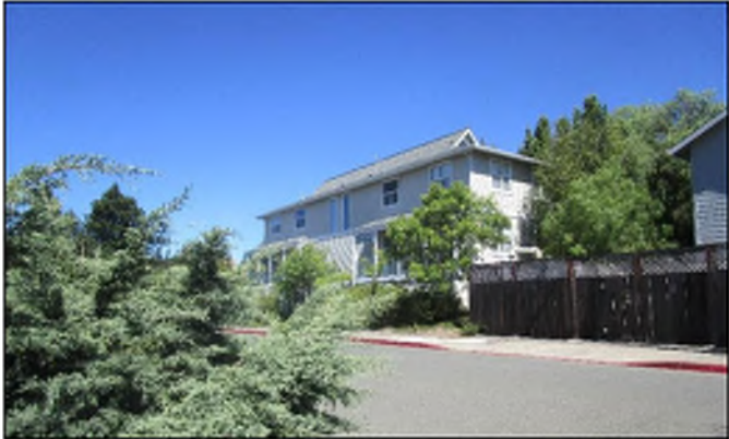
view of south and east
