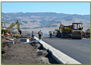
University District Development: Asphalt Paving Operations for New Street Construction.
