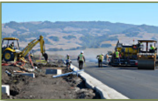
University District Development: Asphalt Paving Operations for New Street Construction.
