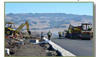
University District Development: Asphalt Paving Operations for New Street Construction.
