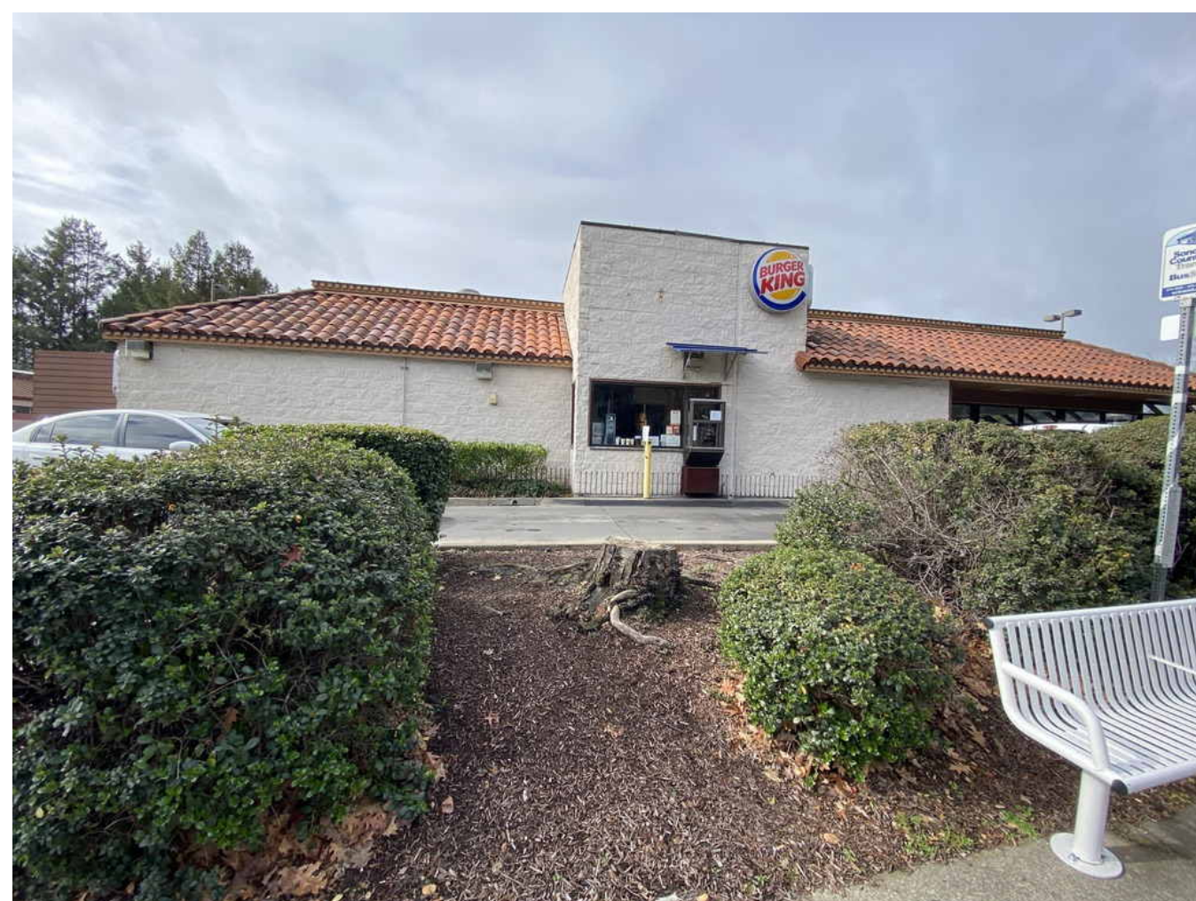
Photo 9: View looking west at the subject property
