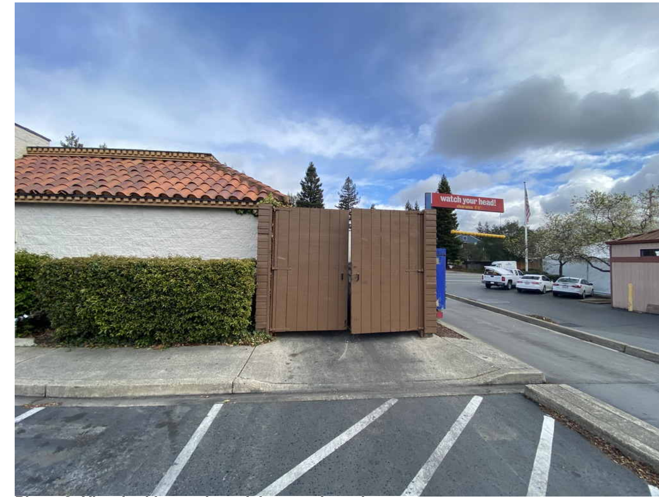
Photo 3: View looking at the existing trash enclosure
