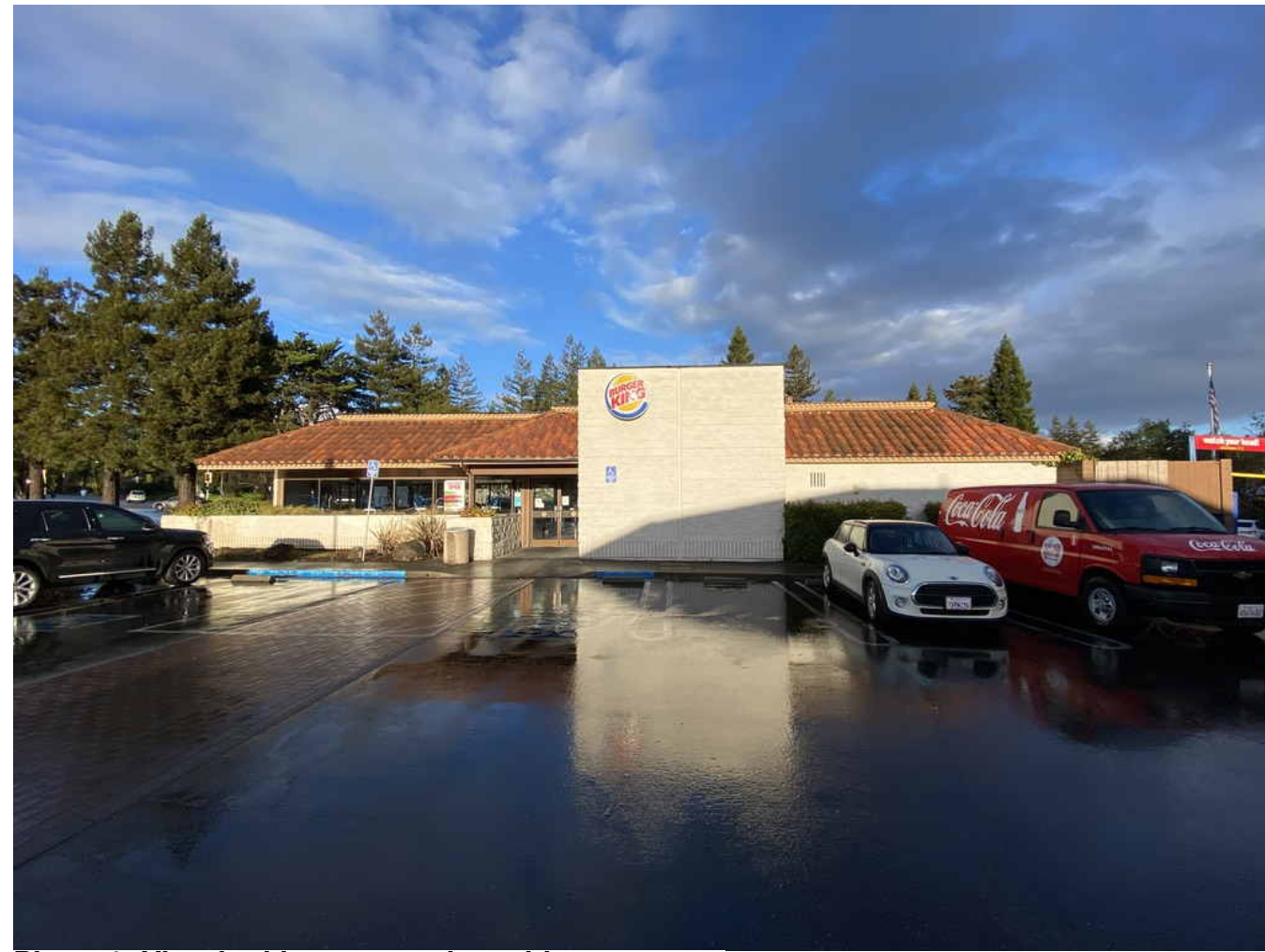
Photo 1: View looking east at the subject property
