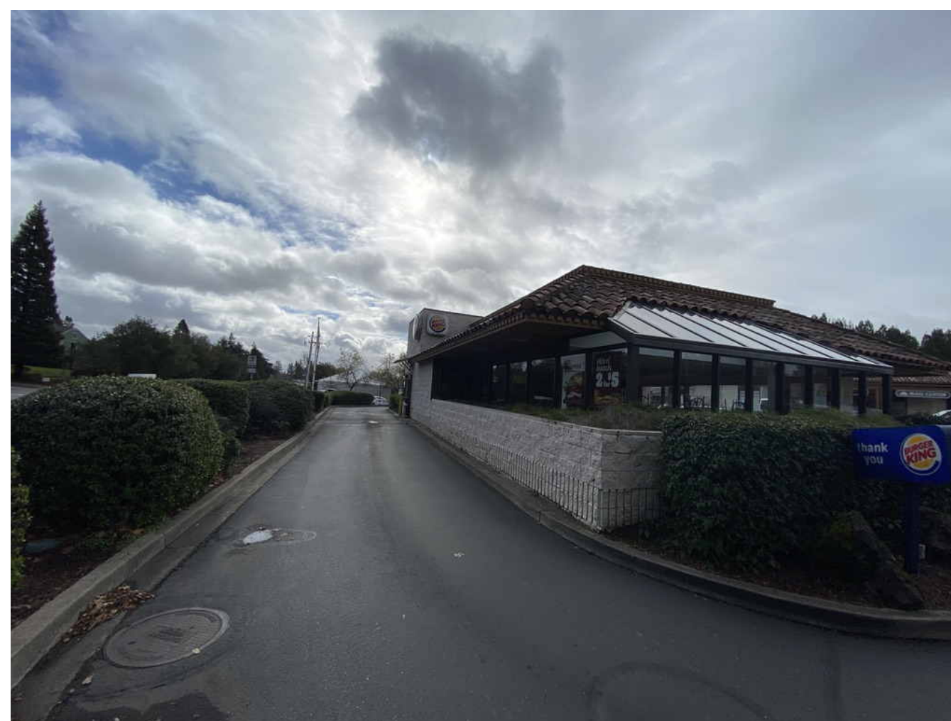
Photo 10: View looking south, towards the drive-thru
